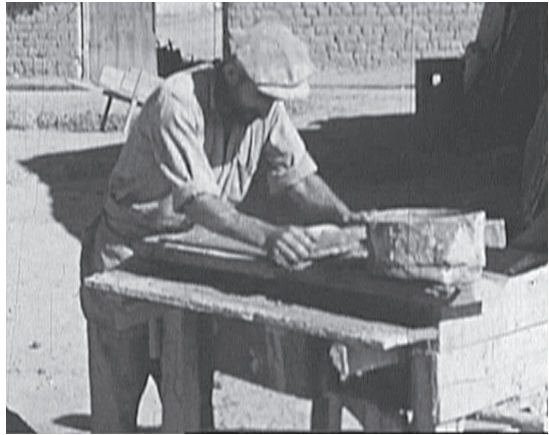
MAKING AND DRYING ROOF TILES. Stills from Triumph Over Time
