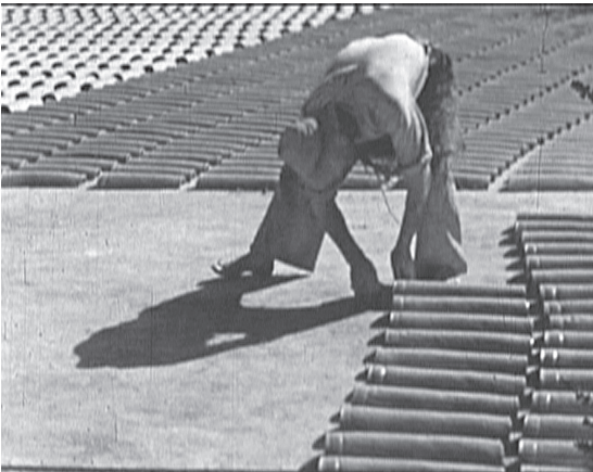
MAKING AND DRYING ROOF TILES. Stills from Triumph Over Time
