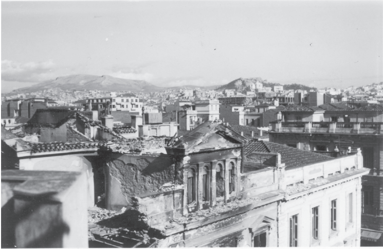
THE DESTROYED ROOFTOPS OF ATHENS IN 1945. From the Gladys Davidson Weinberg Papers, ASCSA
